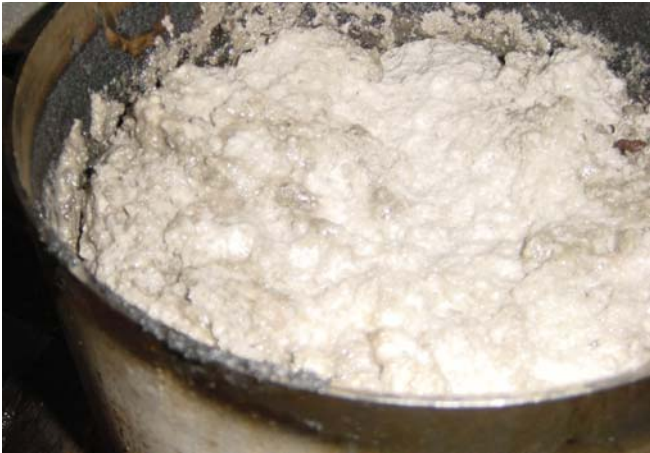
The sludge/refuse chamber of an EBBWCS CD-3-65-1.0
